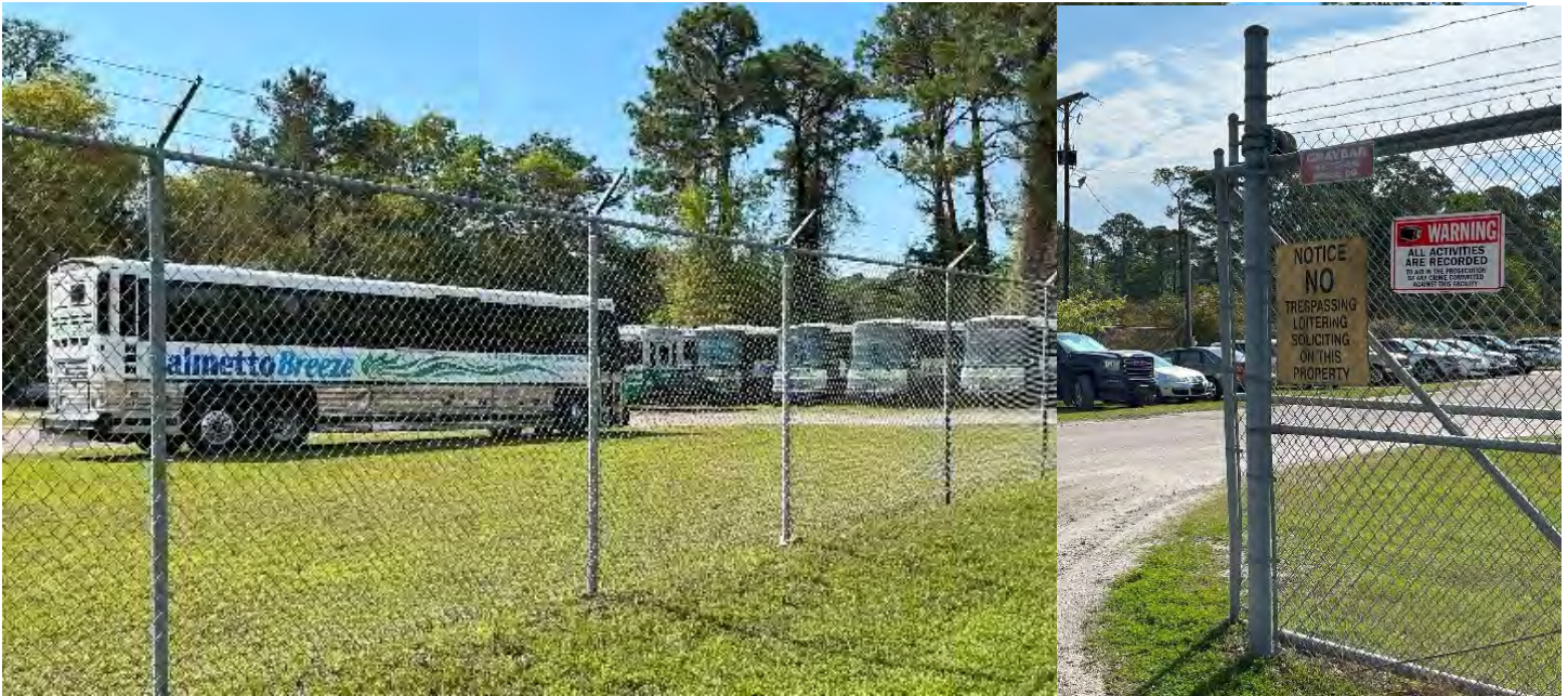
FIGURE 18: BUS PARKING; PALMETTO BREEZE MAINTENANCE FACILITY AND TRANSFER CENTER
